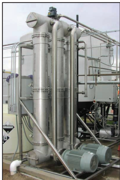
Pall Corporation and Kelitek Engineering partnered to develop a custom system for Hollandia — a fully automated and integrated ceramic membrane-based water purification unit.
