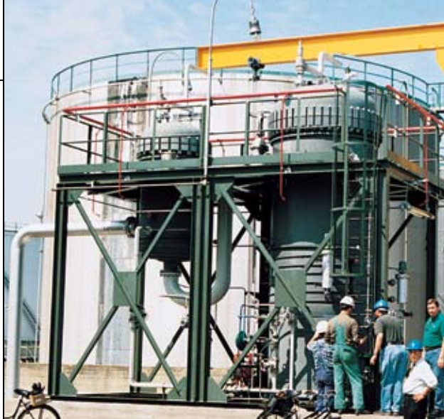
Pall's AquaSep® Plus liquid-liquid coalescer eliminates haze problems from refinery fuels like gasoline, diesel and jet fuels
