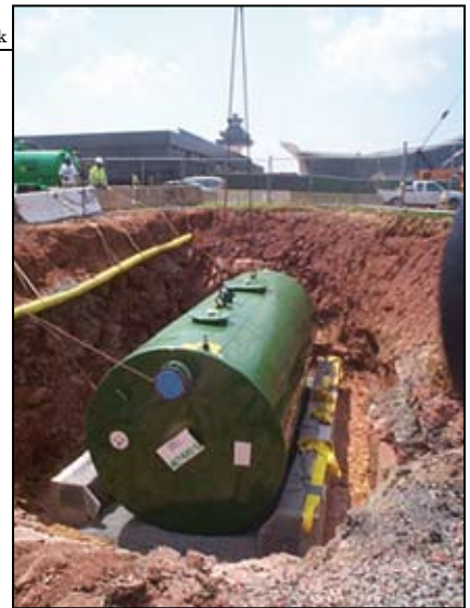
Highland separators with Corella coalescers reduce the level of oil and oil-coated solids discharged by petroleum storage facilities. The Corella inclined parallel-plate coalescers combine the features of both a flat-plate coalescer and a corrugated-plate coalescer into a new self-cleaning design
