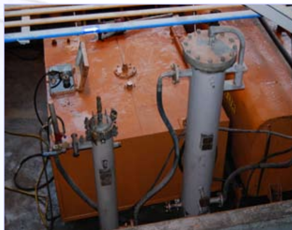
Pall High Flow Ultipleat ® & PhaseSep ® filter housings installed at one of the bulk fuel tanks
