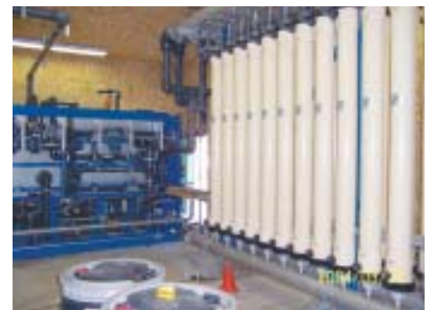
The Kernville, CA, Surface Water Treatment Building.
