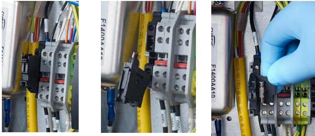
Figure 41: Fuse replacement
