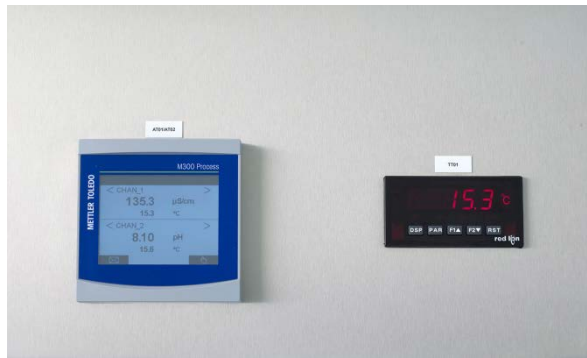
Figure 5.4: pH and Conductivity display (left) and Temperature display (right) Advanced Controlbox
