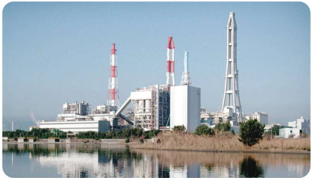
Fig. 3 — Mitsubishi Heavy Industries' 250-MW integrated gasification combined cycle (IGCC) coal-gasification pilot plant for a Clean Coal Power R&D Co. Ltd. initiative containing a porous iron-aluminide ash-filtration system (not visible) from Pall Corp.
