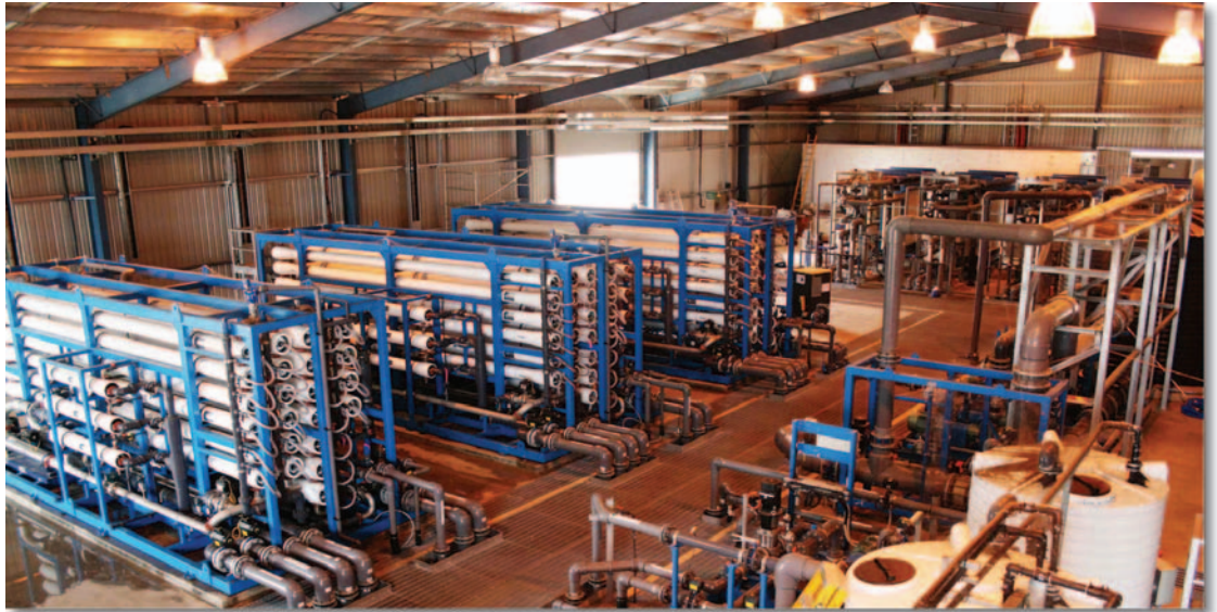
The Pall reverse osmosis systems complete the process of filtering out microbiological and other contaminants.
