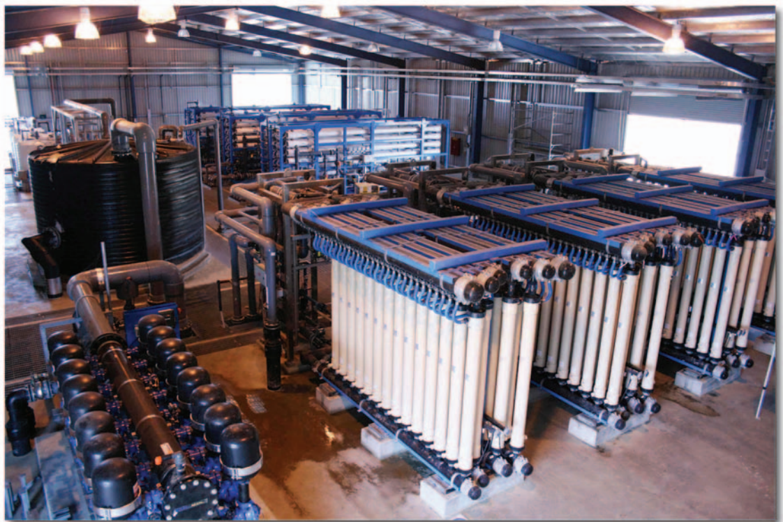
A view of the Pall microfiltration systems (foreground) and reverse osmosis systems.
