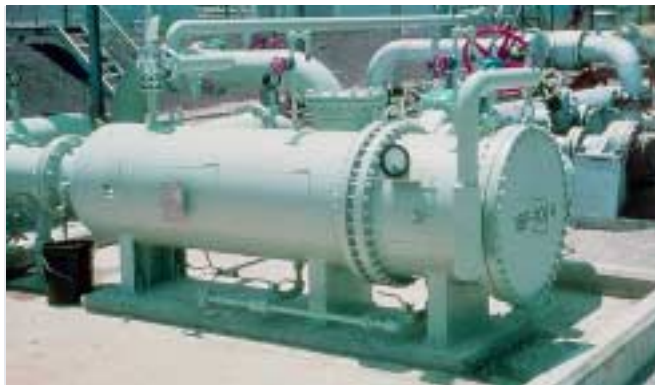
FIG. 2. Installation of the high-flow filter assembly.
