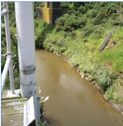
Tangahoe River at intake site – New Zealand
