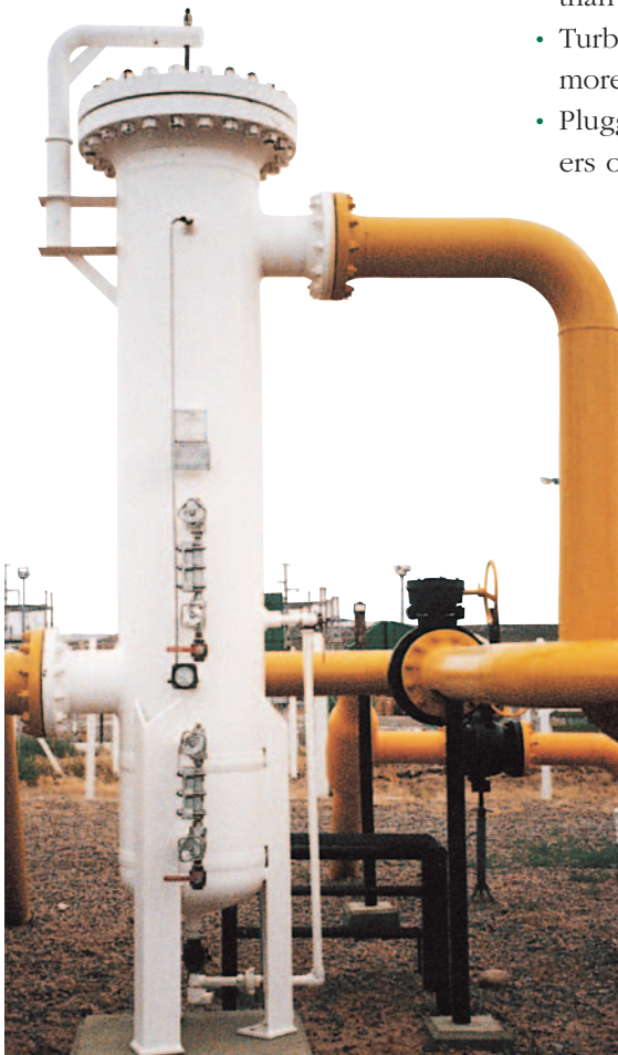
A SepraSol liquid/gas coalescer protects a natural gas turbine from damage caused by liquid aerosols.
