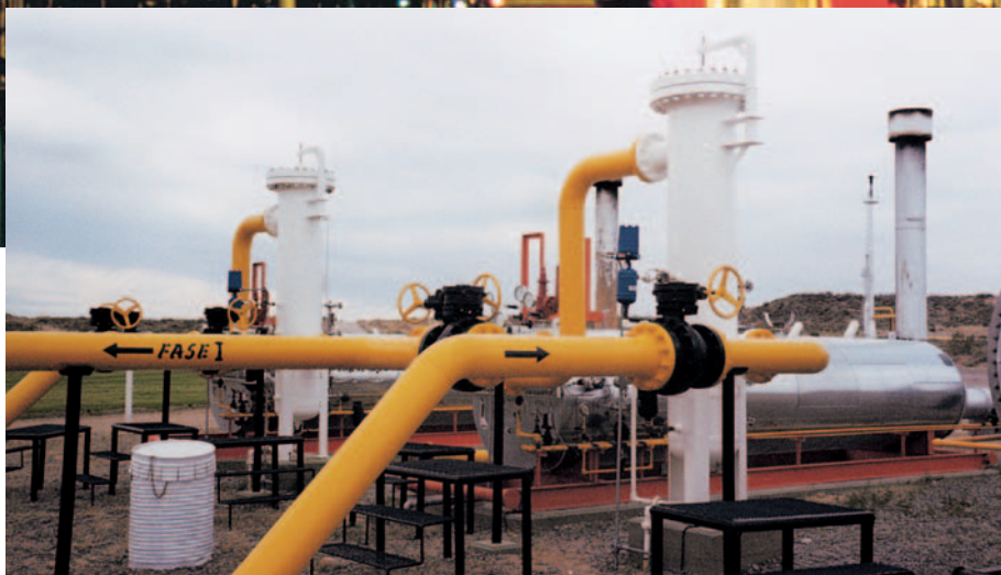
SepraSol liquid/gas coalescer system protecting a compressor.
