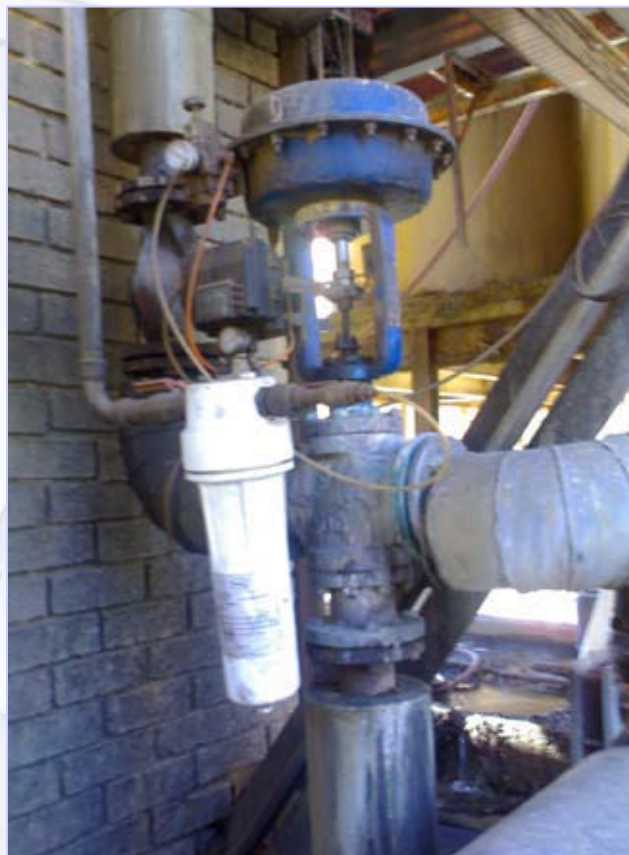
Pall PCY1001G16H13X installed in the Pneumatic System
