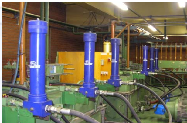
6 x Pall Ultiplex SRT UH319 Series on the pressure line
