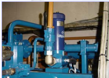
Pall Ultipleat SRT UR319 series filters in the filling and return lines
