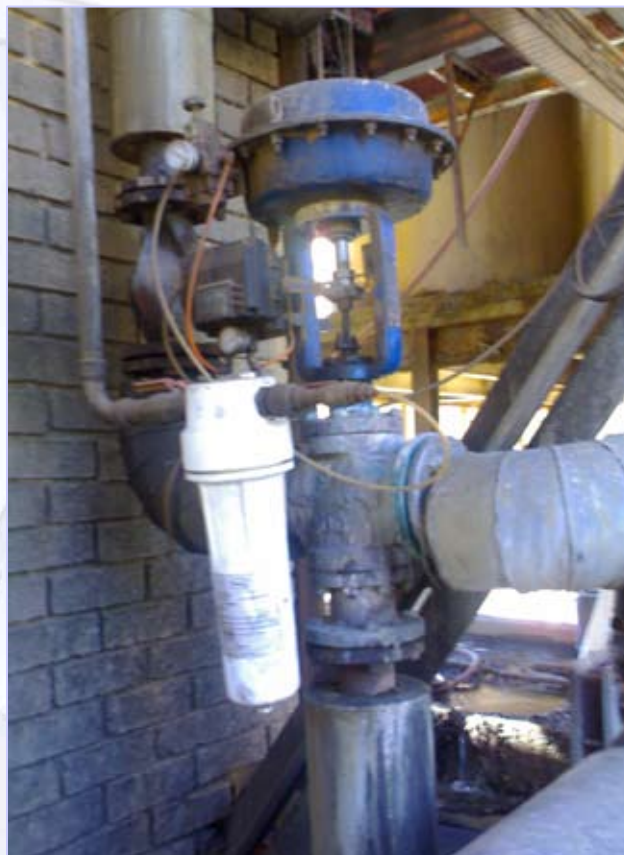
Pall PCY1001G16H13X installed in the Pneumatic System
