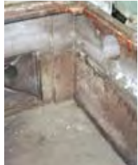
Corrosion in the resevoir
