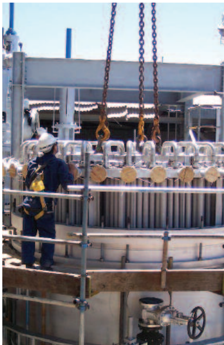
Fig 6: Filter tubesheet assembly installation
