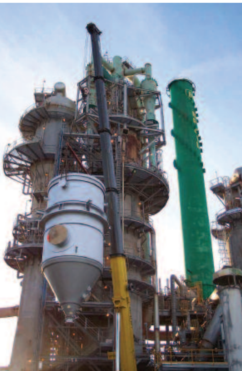
Fig 5: Filter vessel lifted into position
