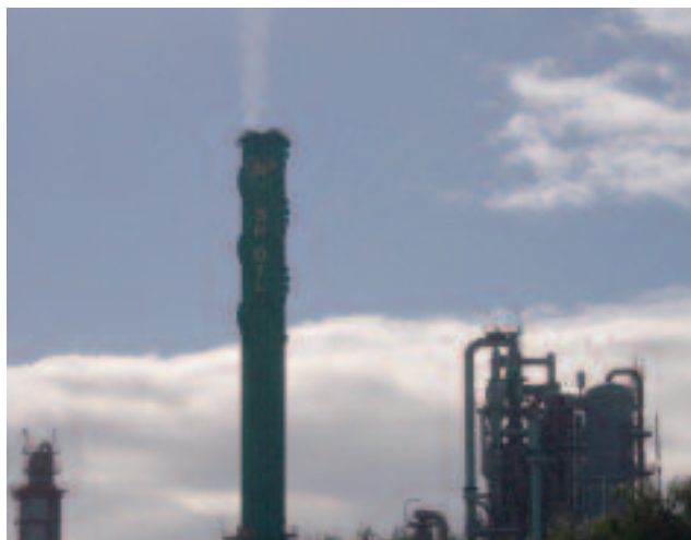
Fig 8: BP RCCU common stack before and after blowback filter start up. (Note: 2 plumes on left hand photo, and 1 plume on right hand side photo).
