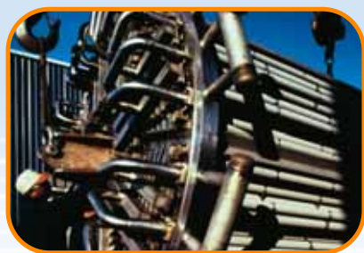
Blowback filter system
