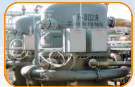
Backwash filter system
