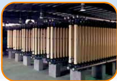
Microfiltration membrane system
