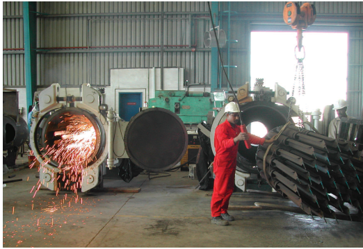
Cut out and removal of existing internals
