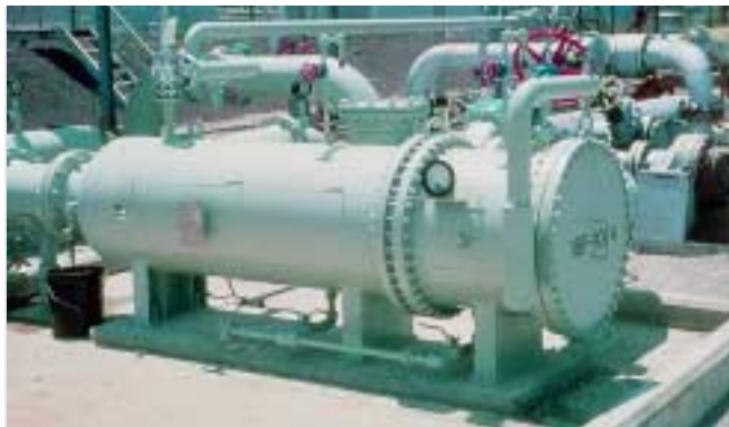
FIG. 2. Installation of the high-flow filter assembly.
