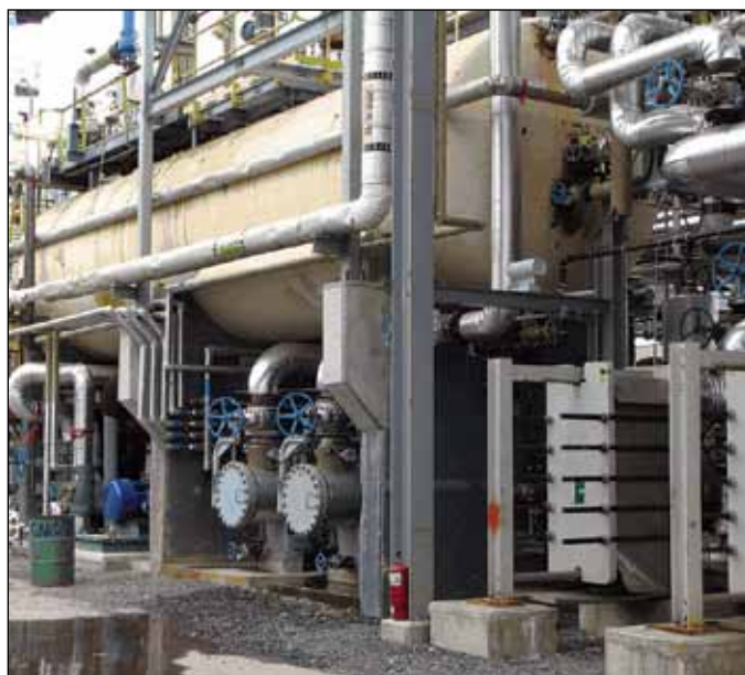
These are duplex Ultipleat High Flow, rich-amine filters (Fig. 6).
