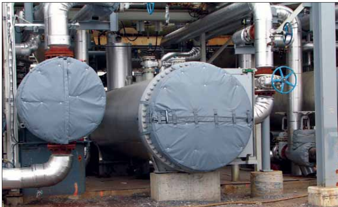
This is a PhaseSep liquid/liquid coalescer unit (Fig. 7).
