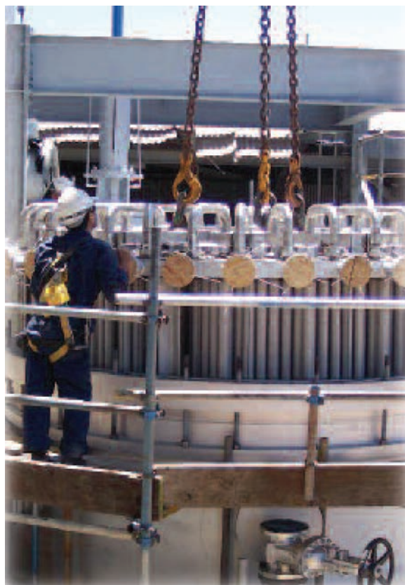
Filter tubesheet assembly installation
