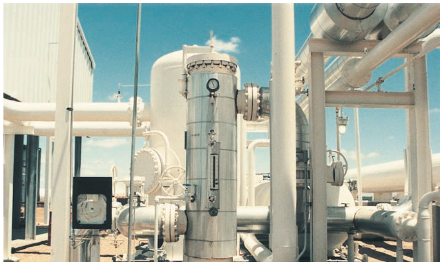
Pall's liquid/gas coalescers remove liquids and solids from hydrogen and fuel gas, protecting turbo machinery and combustion equipment.
