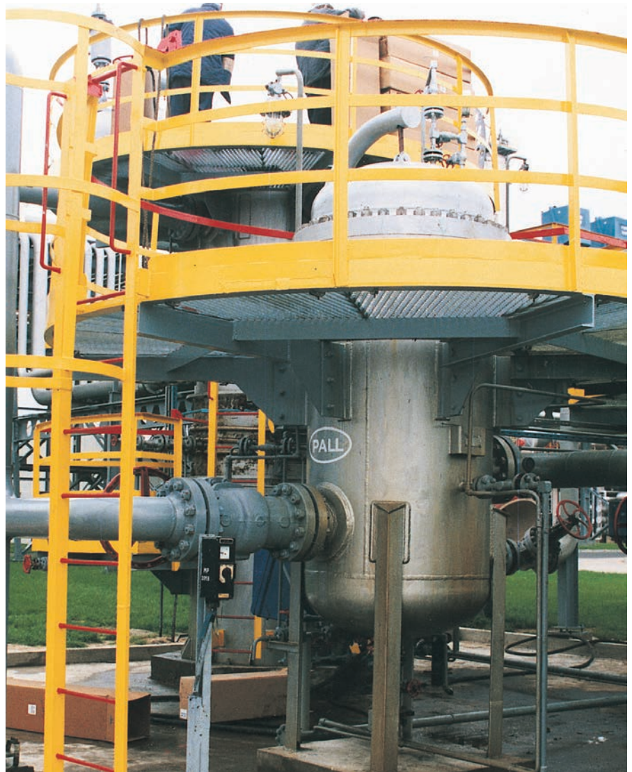
Pall's AquaSep Plus and PhaseSep coalescers are the most cost-effective technology for liquid/liquid separation compared to other methods, including tank settling, electrostatic precipitation, salt drying, sand filtration, and coalescing by mesh pads.
