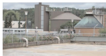
Municipal Sewage Treatment Plant (D): Crailsheim, 5,700 m BRANDOL®
