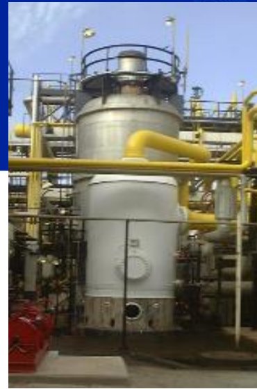
Old separator removed
