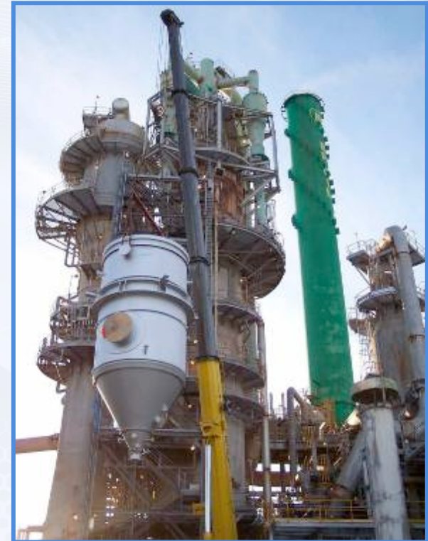
Pall blowback filter systems remove flue gas emissions in refineries
