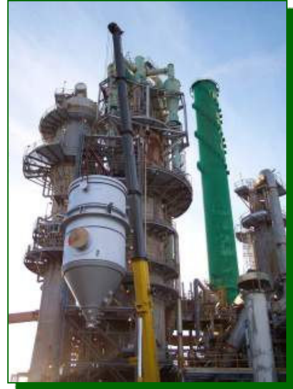
Pall Blowback Filter System used to remove flue gas emissions in refineries
