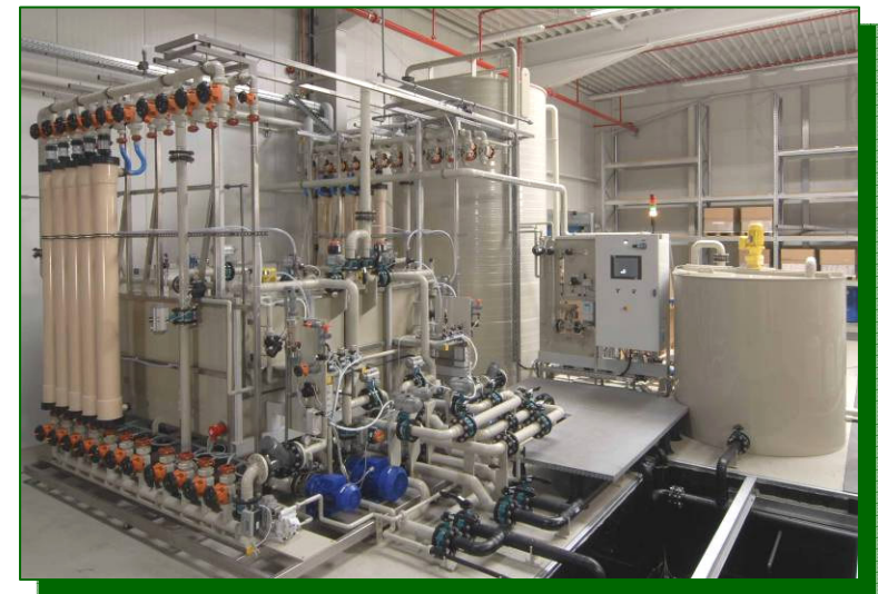
Pall fully-automated, Dynamic Membrane Filtration System, recovers ~95% of DI water used during solar silicon ingot shaping
