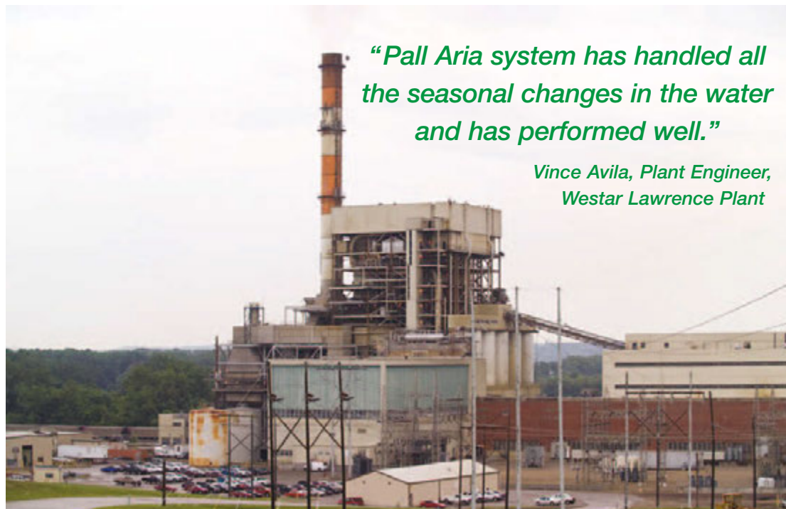
Westar Energy's Lawrence Plant
