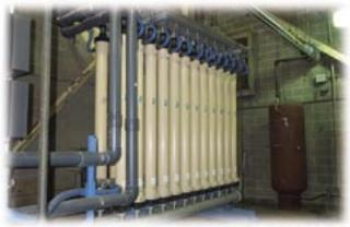
Photo 2. Microfilter module rack.
