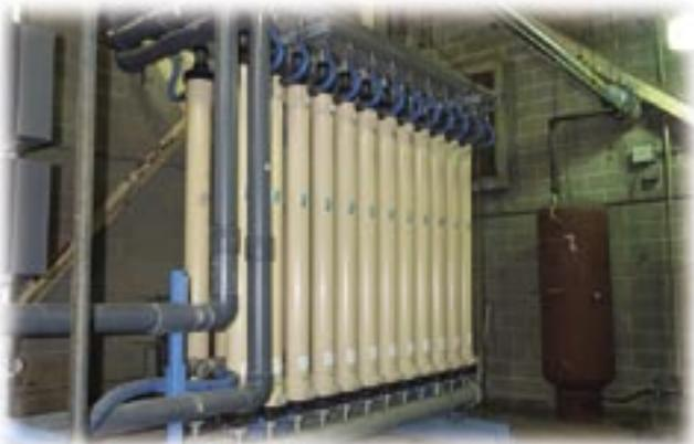
Photo 2. Microfilter module rack.
