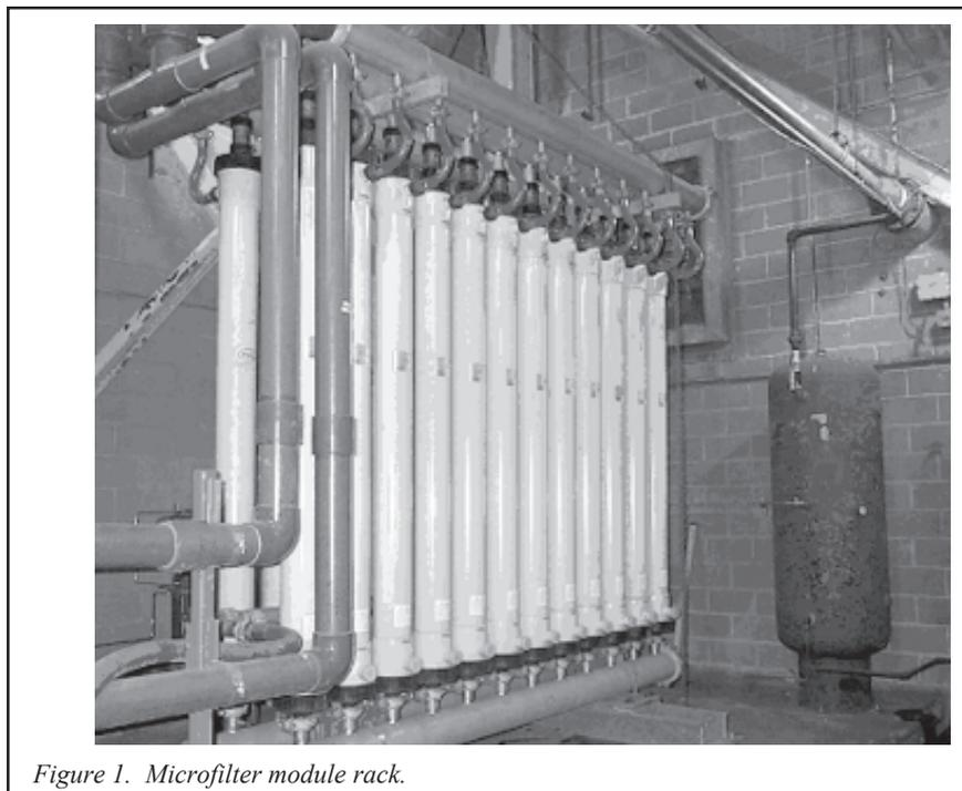
Figure 1. Microfilter module rack.
