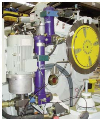
Pall Ultipleat SRT off-loop filter and pump set
