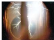
Electrical discharge occurring inside oil tank
