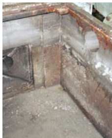
Corrosion in the resevoir
